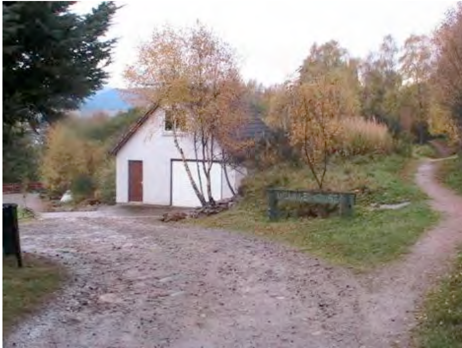
Fig. 13- Showing section of path that would need upgraded to track to access single house (immediately behind garage) at western side of site.
